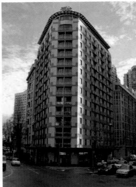
Southern Cross Suites, has been purchased by leading timeshare group Trendwest South Pacific, in a deal that opens the way for a change in the Sydney apartment and hotel market
